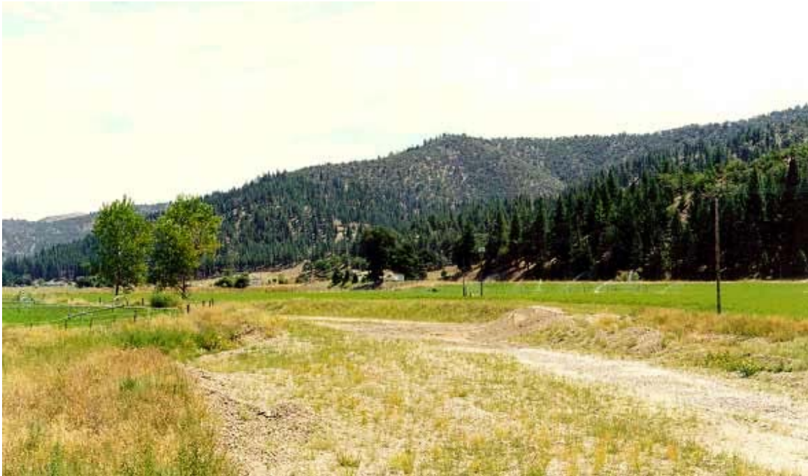
Figure 9. The Moffett Creek channel lacks definition and riparian trees because of drops in the groundwater due to pumping. The stream was once perennial and harbored coho salmon.
